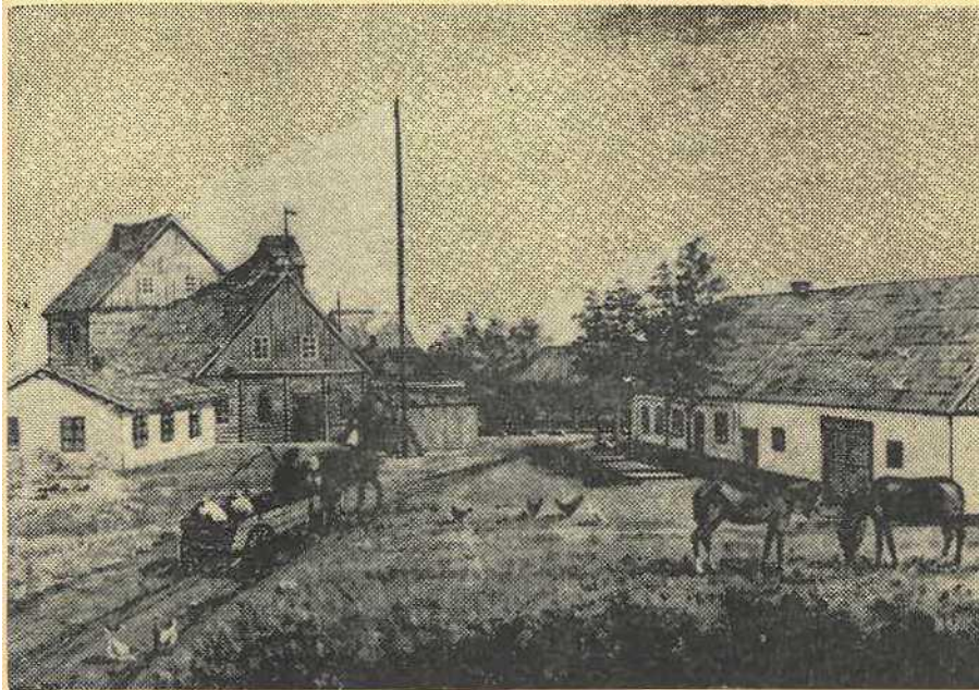
Eckert's mill in Kamyshovoye
